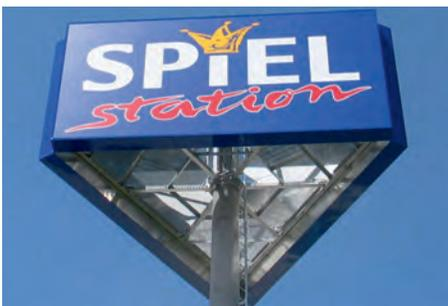
**MATERIAL** Substructure made of hot-dip galvanised steel
