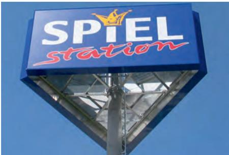
**MATERIAL** Substructure with accessible maintenance platform made of hot-dip galvanised steel
